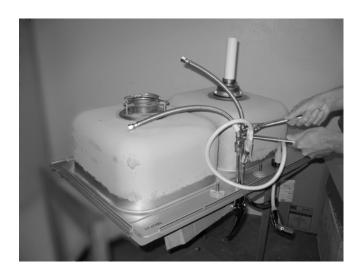
3. Connect the continuous waste assembly to the strainers. If you're installing a food disposal, this step will have to wait until the sink is mounted in the countertop. But if you just have 2 strainers, it's easier to assemble the drainage plumbing interconnecting the two bowls before the sink is installed in the countertop.
