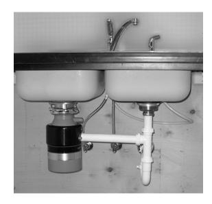
7. Remove the aerator from the faucet. Turn the faucet to the full "On" position and open both supply valves fully to flush the lines of any debris. Check for leaks in both the supply lines and drain pipes while the water is running and after it is turned off. Reinstall the faucet aerator.
